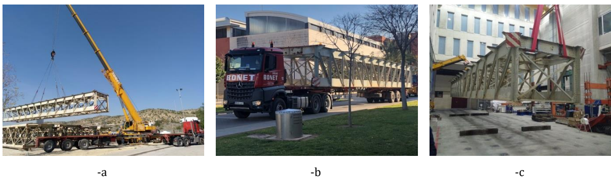
Figure 8: Movement phases: taking from storage area (-a), movement (-b) and laboratory placement (-c).
