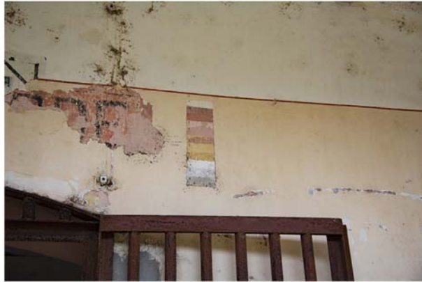
Figure 1 Excavated paintwork at the Camp de la transportation, Saint Laurent du Maroni (June 2018). Photo with kind permission of Claire Reddeman.
