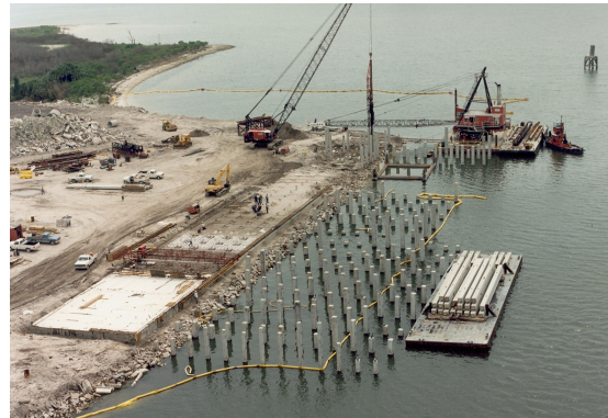
(b) Harbour structure foundations
