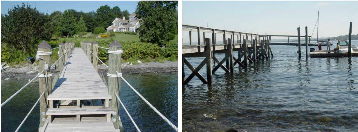
Figure 3. Typical wood-framed docks and floats sampled in this study.
