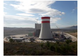
Fig. 3 The Greek Ptolemaida V 615 MWe power station (under construction)
