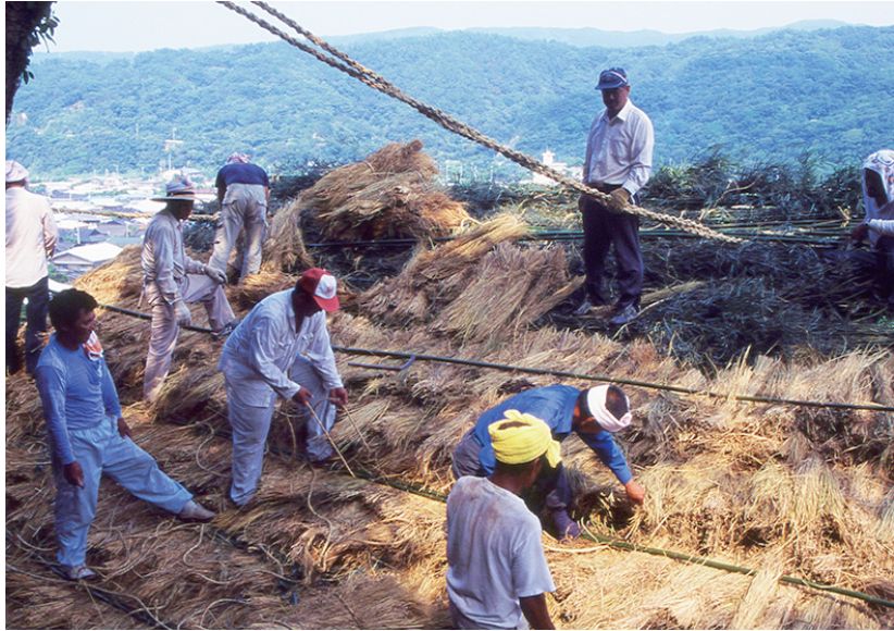
FIGURE 41. Making a thatched, single-roof hut (lean-to) for the Shochogama festival/handing down thatching technology, Sept. 1994.
