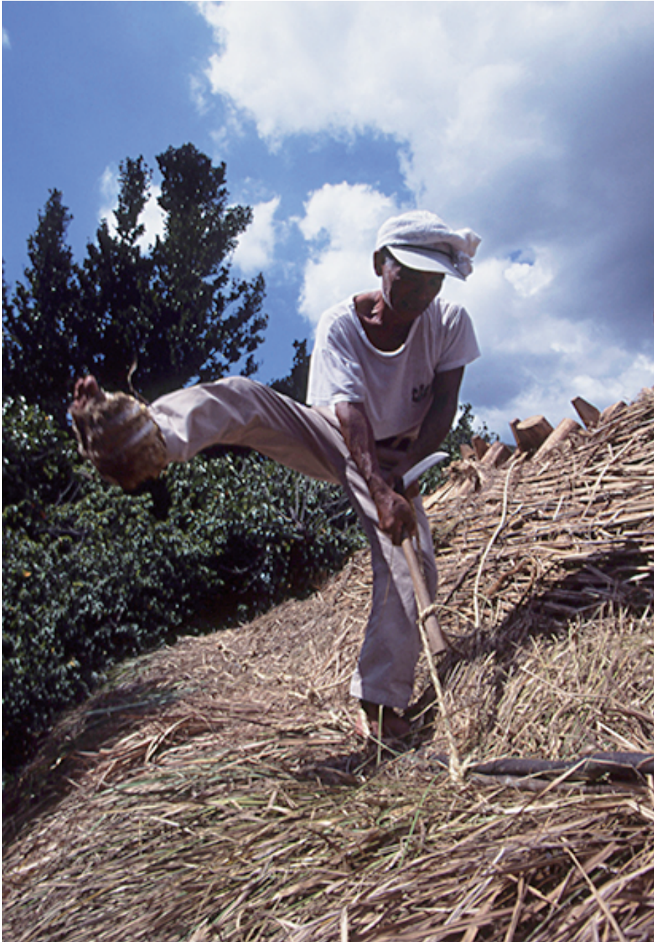
FIGURE 23. Wrapping a straw rope around the leg and stepping on it with full power to tighten the thatch, March 1995.
