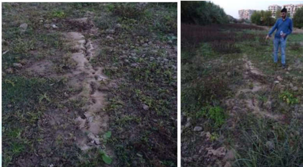
Figure 9. Images of the liquefaction phenomenon and sand boiling in different parts of the riverbed near Shahid Shiroodi Mehr housing complex (IIEES, 2017).
