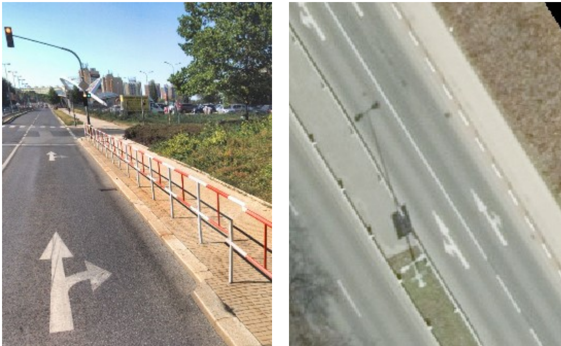
Figure 50: Protective metal railing with bright red and white paint; from driver's perspective (left) and in aerial image (right)
