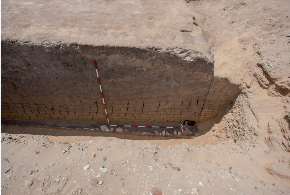
Fig. 19 Northern wall and north-western corner of AS 104, standing on the platform, view from the north (photo M. Peterková Hloučová)
