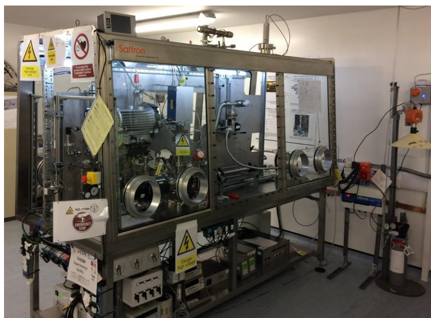
Fig. 1. Plasma exposure system after inactive gas commissioning. The system is partially built into the secondary containment system which will be required for tritium commissioning.
