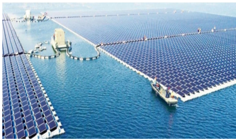
Figure 1. Floating solar power plant (Source: Brandon, 2017 [23]).
