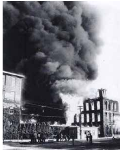
Manville Mill, Largest fire in Rhode Island, September 12, 1955
