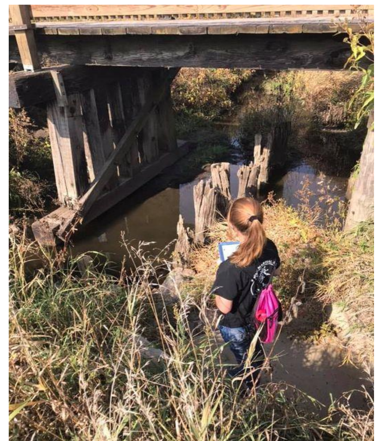
Figure 2. Views of the Middle Site.
