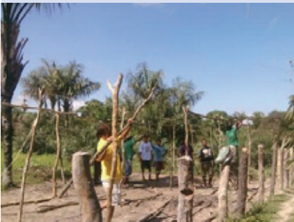
Photograph 01 – Plant nursery construction
