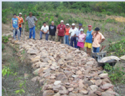
Photograph 02 – Collective activity for construction of succession dam
