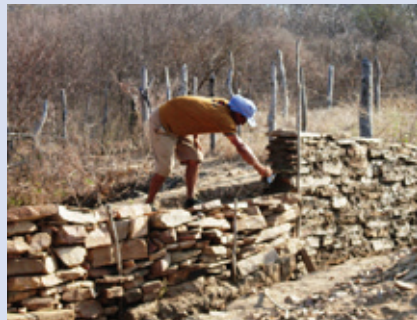
Photograph 02 – Construction of dry stone dam
