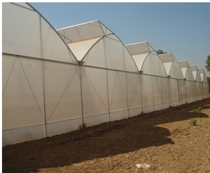
Metal greenhouses in Jamaica (Photo: Isratech Jamaica Ltd.)
