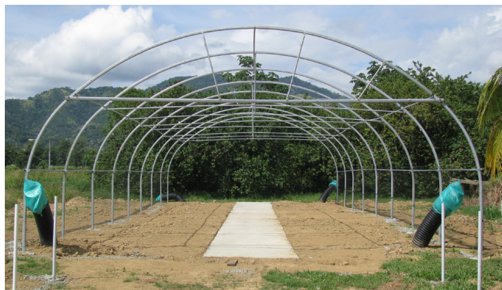
GIFT tropical greenhouse, under construction. (Photo: CARDI/UWI)
