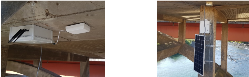
Fig. 10. Sensors installed on Original Structure
