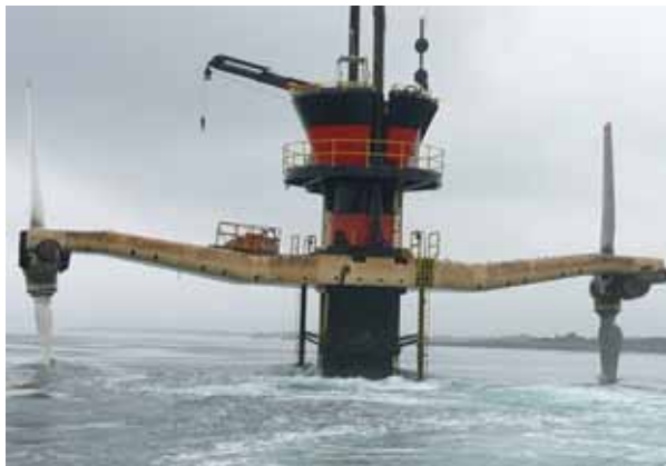
Figure 1. The wake downstream of a Marine Current Turbines Ltd tidal turbine, raised out of the water for maintenance. Source: "Frazer-Nash Irons SeaGen Wrinkle," renews , 5 March 2014, http://renews.biz/62085/frazer-nash-irons-seagen-wrinkle/ (accessed 23 July 2018).
