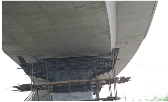
Fig. 9 – Reinforcement and reconstruction of bridge piers
