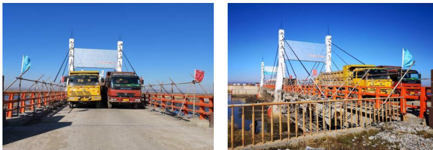
Fig. 7 - On-site loading situation
