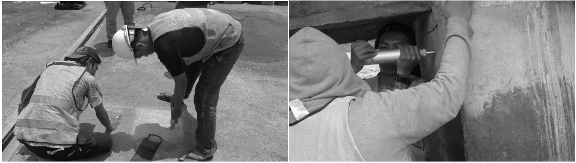
Gambar 4. Proses Pengujian Hammer Test
