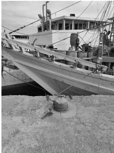
Gambar 5. Bollard Pelabuhan Paotere Makassar (Survey)
