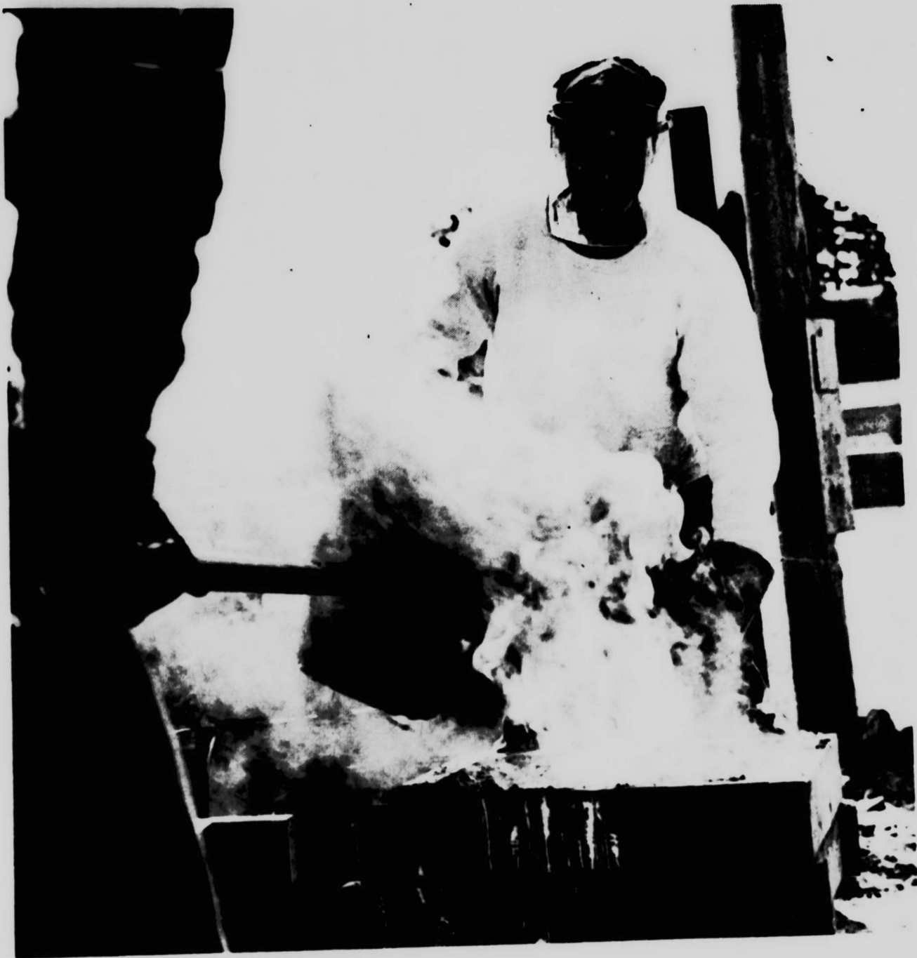
After the pieces of styrofoam are invested in sand the bronze is carefully poured into the form.
