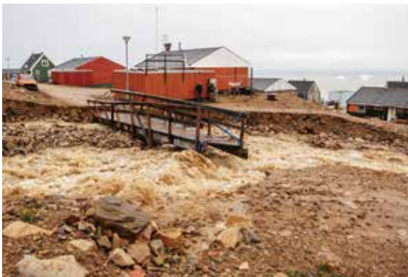
Fig. 9-4: A bridge destroyed by a flooding river flowing from a glacier near the village of Qaanaaq (photo by S. Sugiyama, Greenland).
