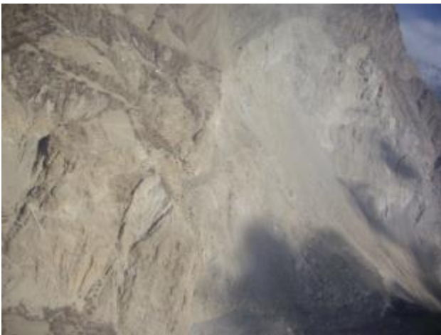
Figure 4: An aerial View of Attabad landslide, Source: FOCUS Pakistan, according to the interpretation of the features developed after the landslide, the landslide event occurred in 3 stages. First the central eastern portion came down as result the left portion came down due to dragging force and at the third stage; upper rock ridge came as observed at the top of the clay deposits above the debris mass. Minor time difference anticipated between the 1 st and 2 nd
