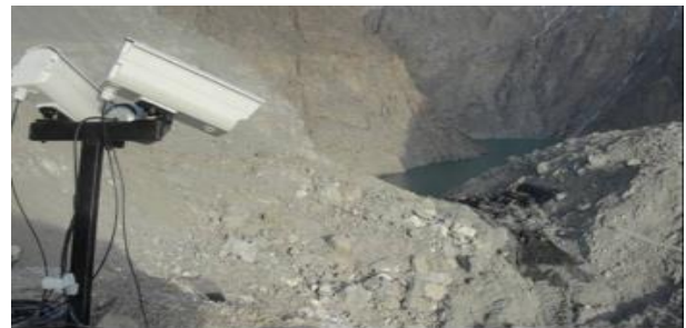
Figure 8: CCTV cameras installed at the
