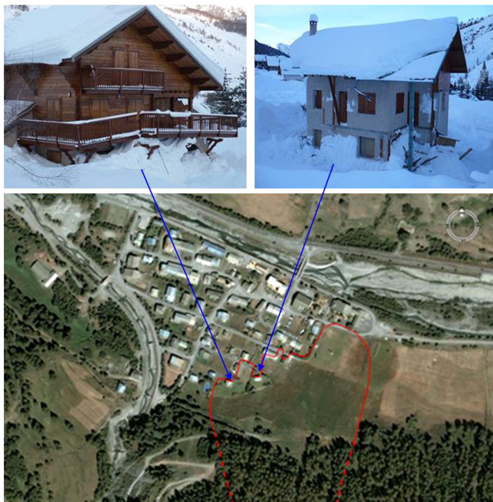
Fig. 2. Avalanche in Ristolas, December 16th 2008. La Combette avalanche path, Queyras massif, France. Avalanche flow path and runout area are marked with a red outline. Two houses were hit and damaged (upper panels). Several people were buried outside the houses, but were rescued. Pictures M. Deschatres/Cemagref.
