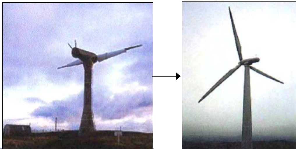
Fig. 2.6 (a) The old model of biggest 3 MW wind machine which was dismantled and replaced with modern 2 MW wind machine (b) [16]
