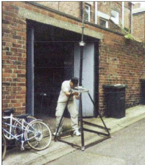
Fig. 6.5 Shaft and Shaft supporter on pre-assembling the wind machine
