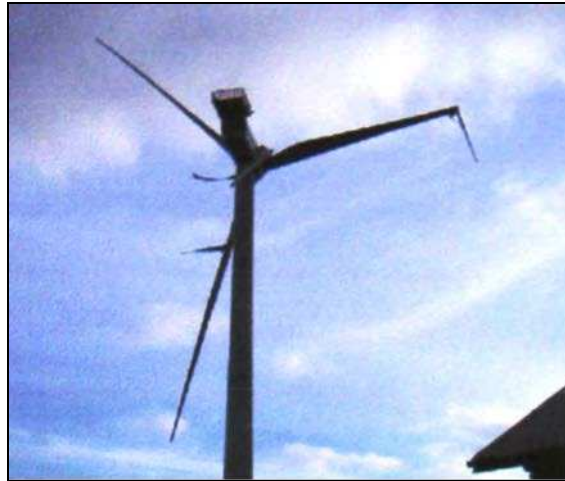
Fig. 2.5 The damaged 2 MW wind machine which is located at Tjaereborg in Denmark [15]
