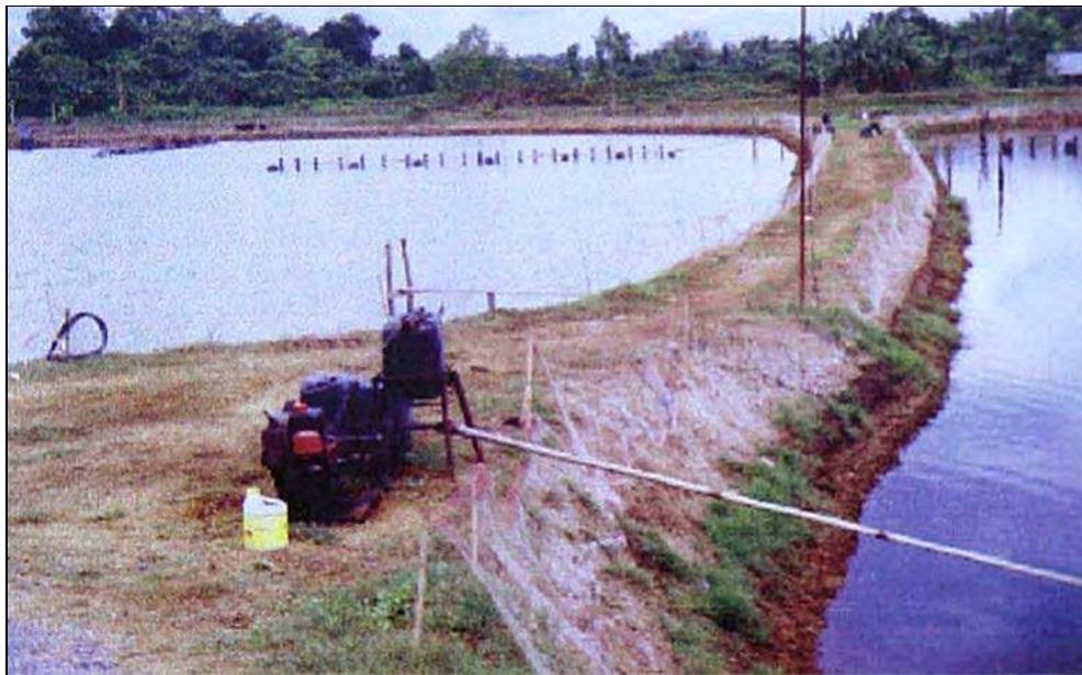
Fig. 6.33 Two-stroke diesel engine for conventional water treatment
