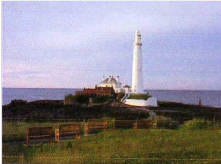
Fig. 6.12 The site before wind machine instillation at St Mary's Island
