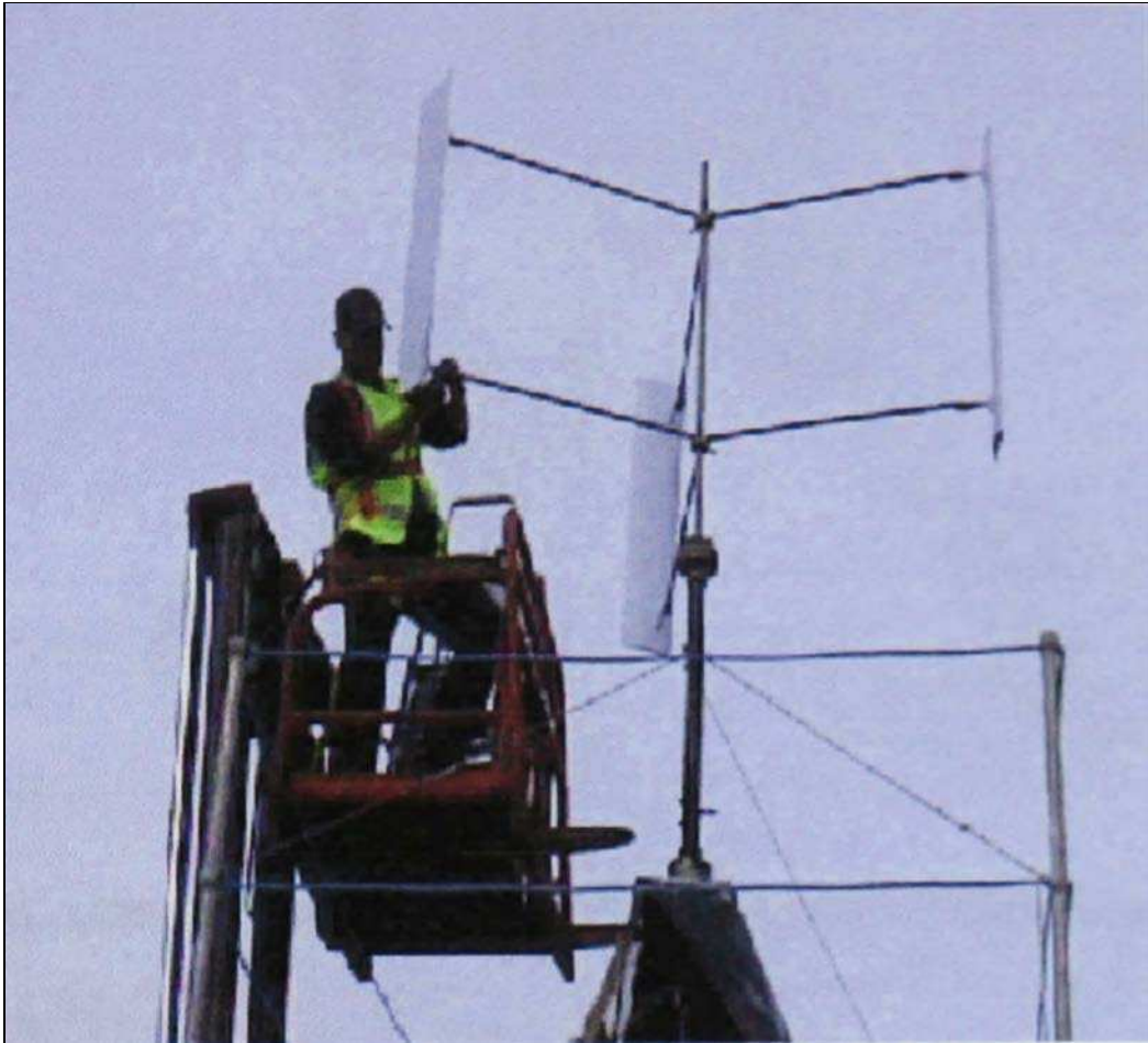
Fig. 6.24 Folk lift used for assembling the rotor to the structure
