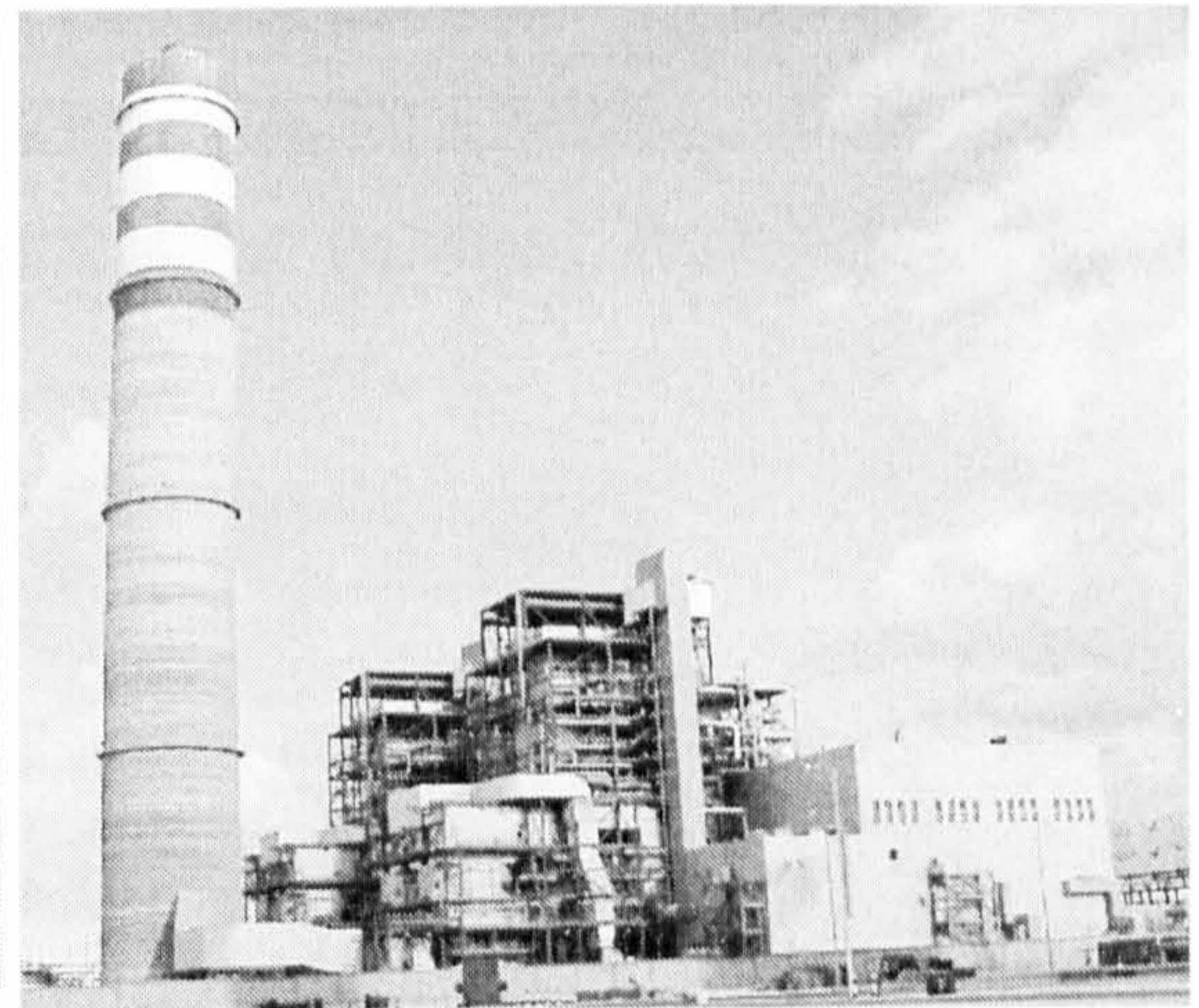
Figure 47-b Sidi Krir Power Station
