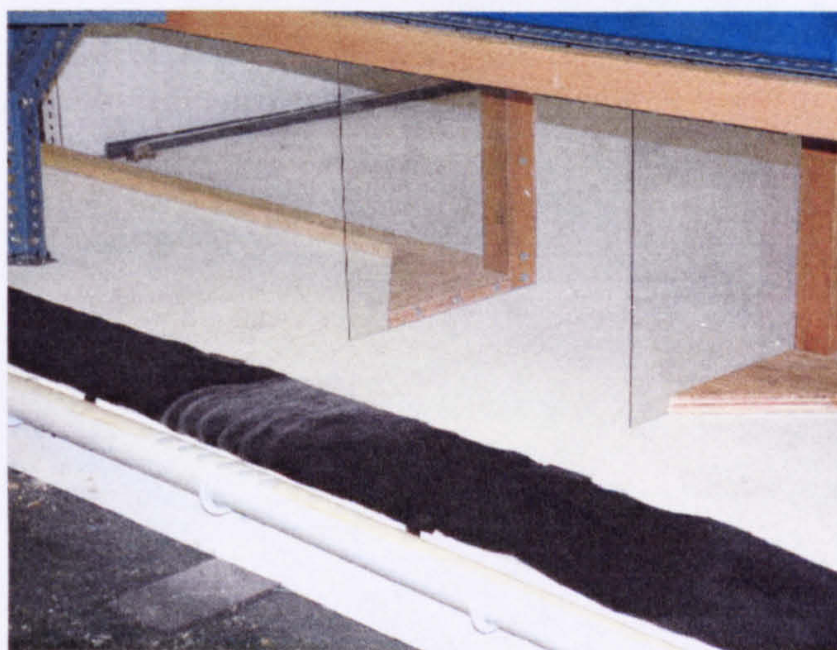
Figure 5.21 - Piping arrangement used to deliver smoke to the vicinity of the inlet
