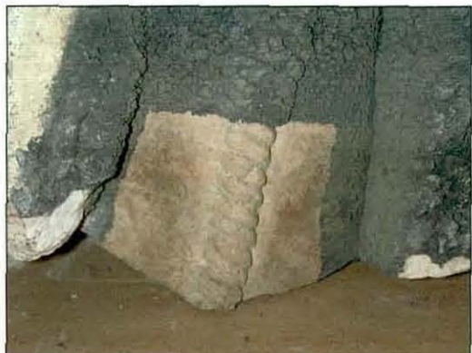
Figure 1. Laser cleaning of stone gargoyles (After Agapaki [7] )
