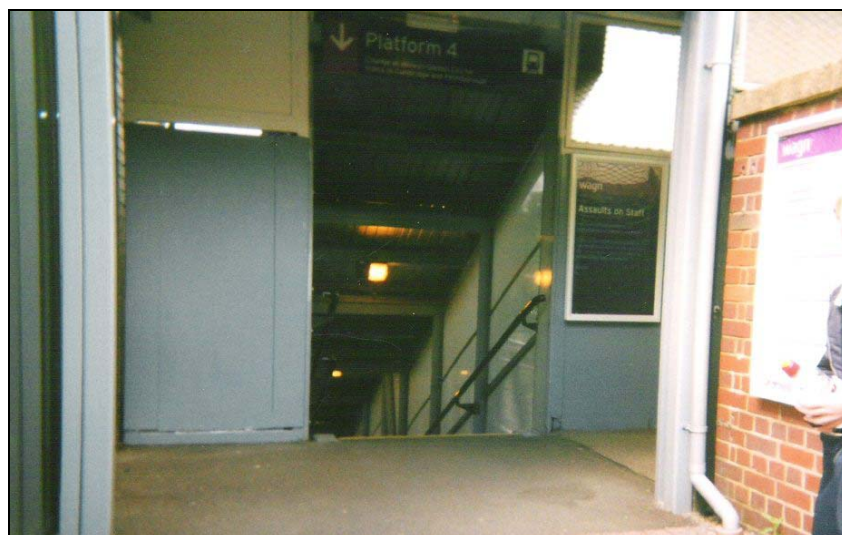
Figure 10.11 Photograph of the train station
