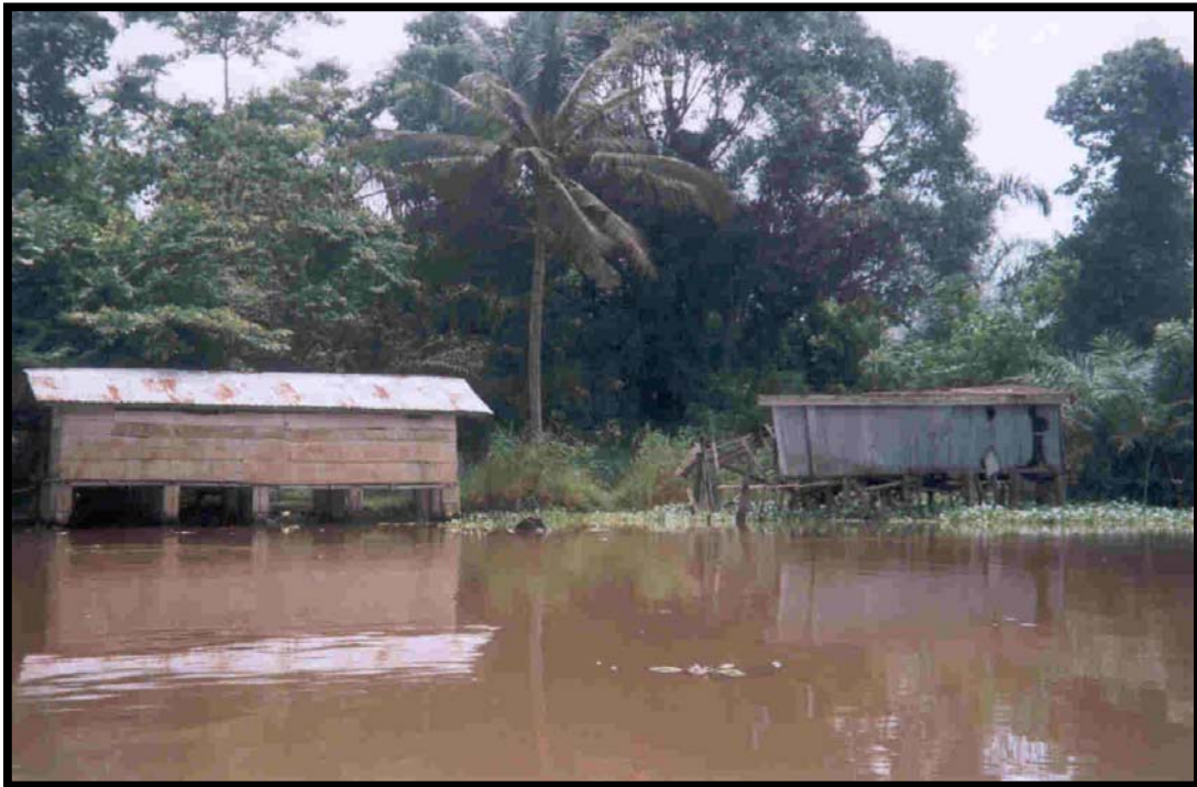
Figure 7. 5 Over-hung toilets by the Elebele / Otuoke Creek
