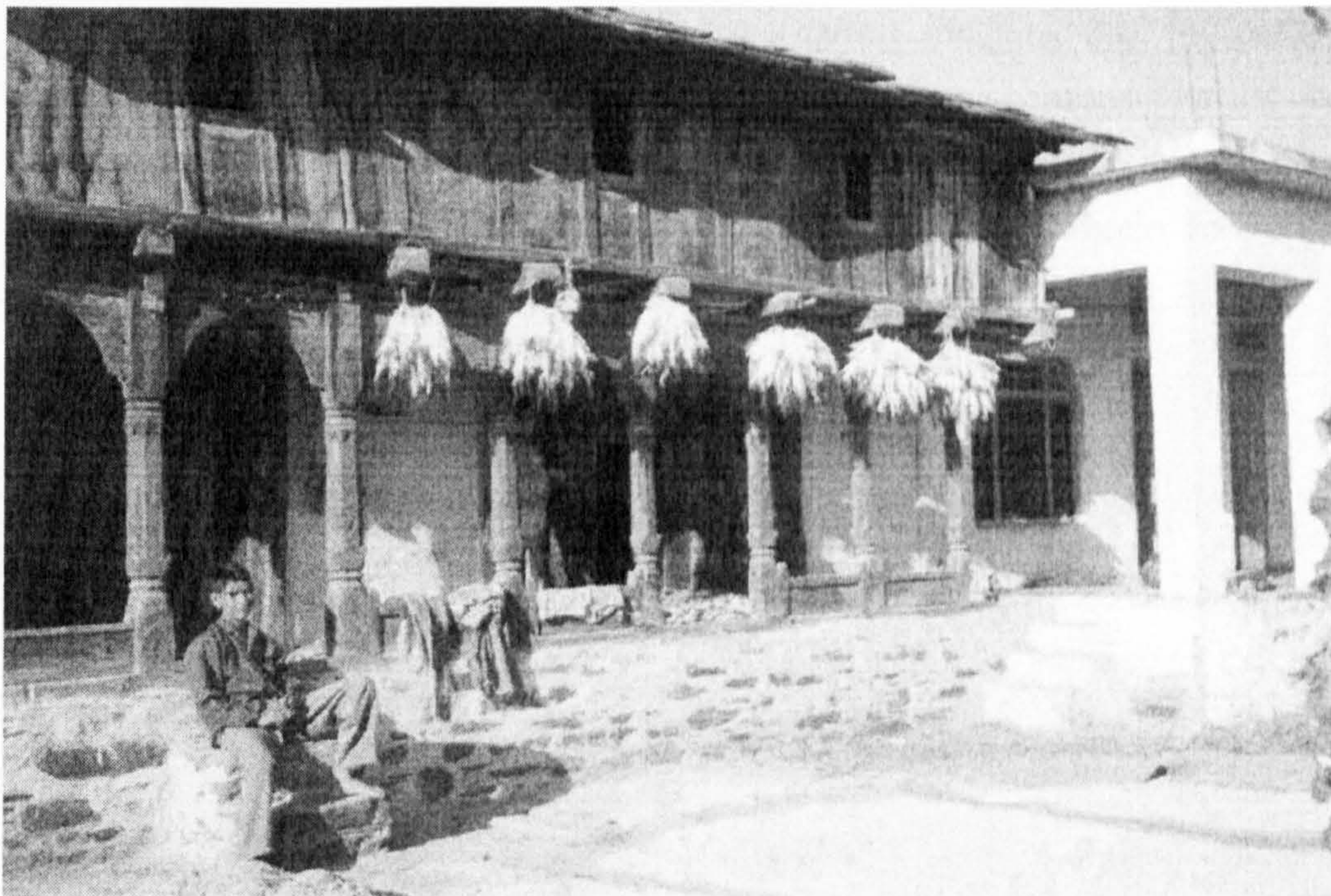
Photograph 3.1. A house with traditional architecture in a remote Tehri village
