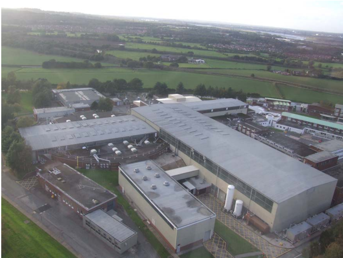
Figure 7.9 Daresbury Laboratory synchrotron radiation source and experimental hall buildings
