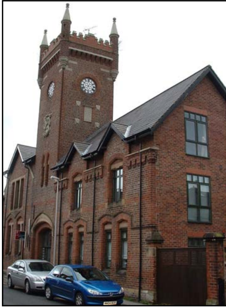
Figure 5.2. The Drill Hall, with T. U. Brocklehurst's clock tower.
