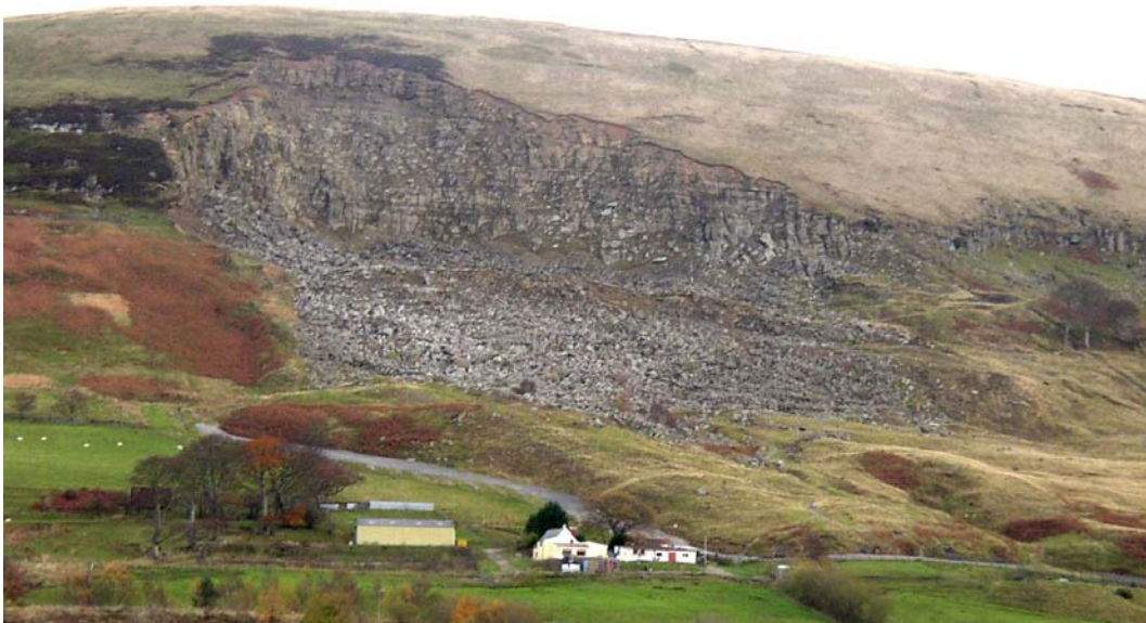
Figure 6.1. The East Pentwyn landslide.
