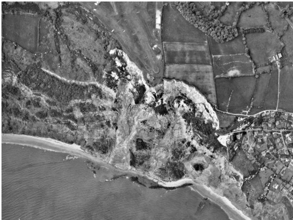
Figure 2.9. Aerial photograph of the Black Ven landslide (UK) showing distinct features of a mudslide system (Ordnance Survey: © Crown copyright).
