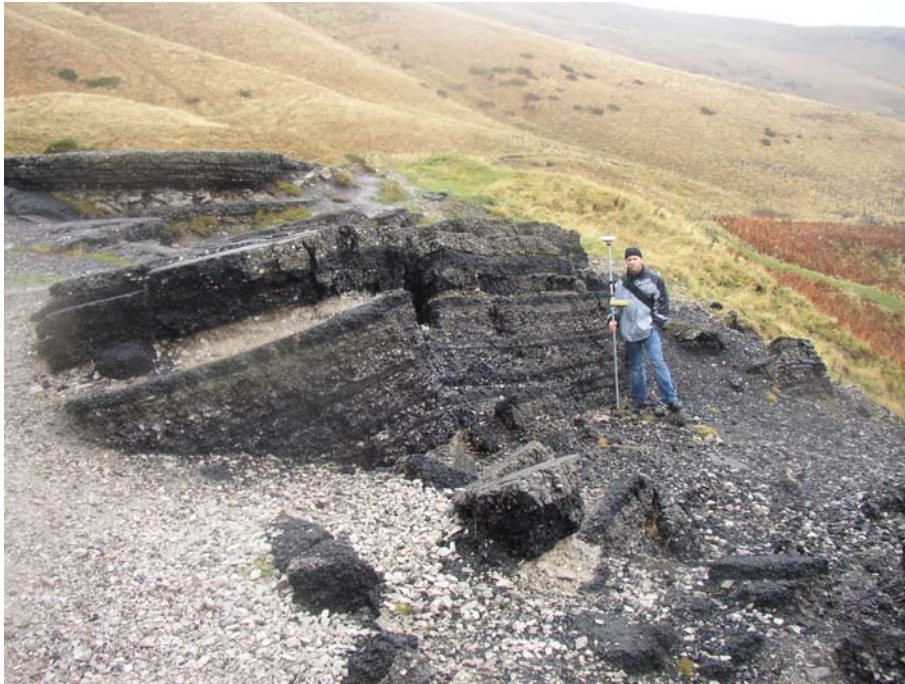
Figure 5.5. Thick layers of tarmac, exposed in the upper road section.
