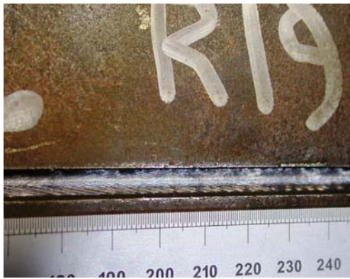
a) weld (run) No. 19
