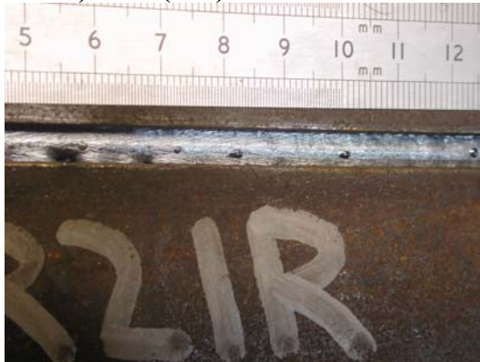
d) weld (run) No. 21
