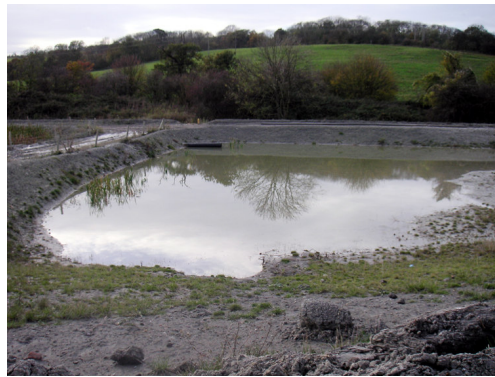
Figure 3-4. Brogborough landfill. A lagoon dug to contain surface water run off. The water is monitored quarterly for presence of leachate and other harmful chemicals (23 rd February 2005).
