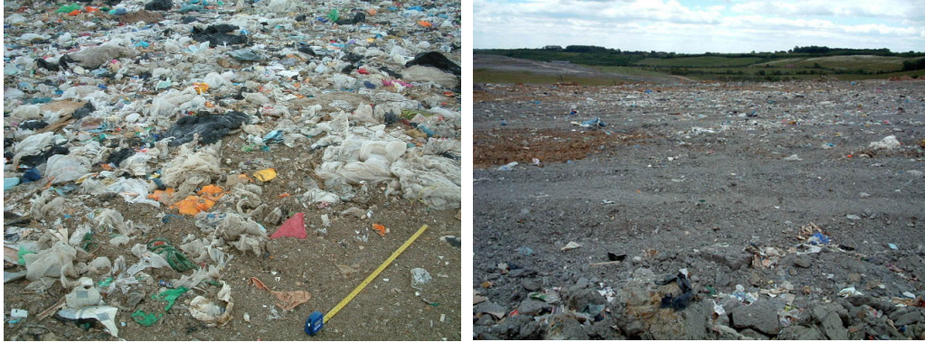
Figure 3-6. Brogborough landfill. Left: waste deposited and immediately compressed in the open cell. A one-meter length is shown in the image. Right: temporary layer of clay deposited on top of the tipping area to cover the waste (09 th May 2005).
