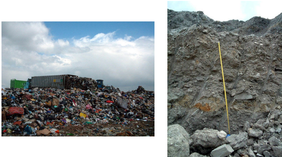
Figure 3-8. Brogborough landfill. Left: batter of an open cell. Right: high vertical step in an area where the daily clay is piled and managed. A two-meter length is shown in the image. (09 th May 2005).
