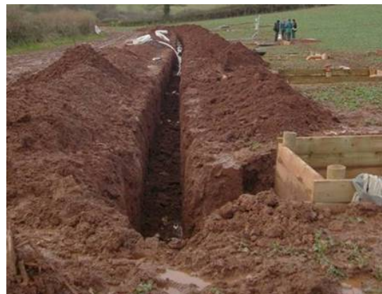
Plate 3.1-2 Pit drainage channel (Tivington)
