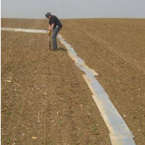
Plate 3.1-3 Bunding installation. Source www.sowap.org
