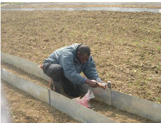
Plate 2.1-5 Installation of erosion plots
