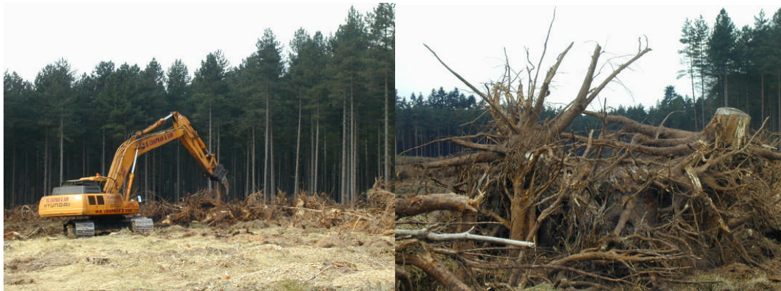
Plate 1.2 De-stumping of clear-fell site at Thetford forest, East Anglia. April 2003
