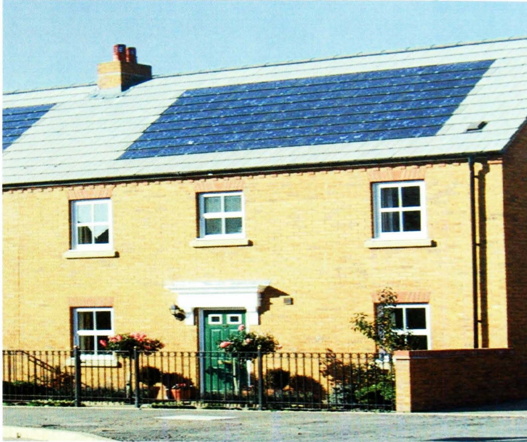
Figure 5.4 Roof-integrated PV tiles in private development
