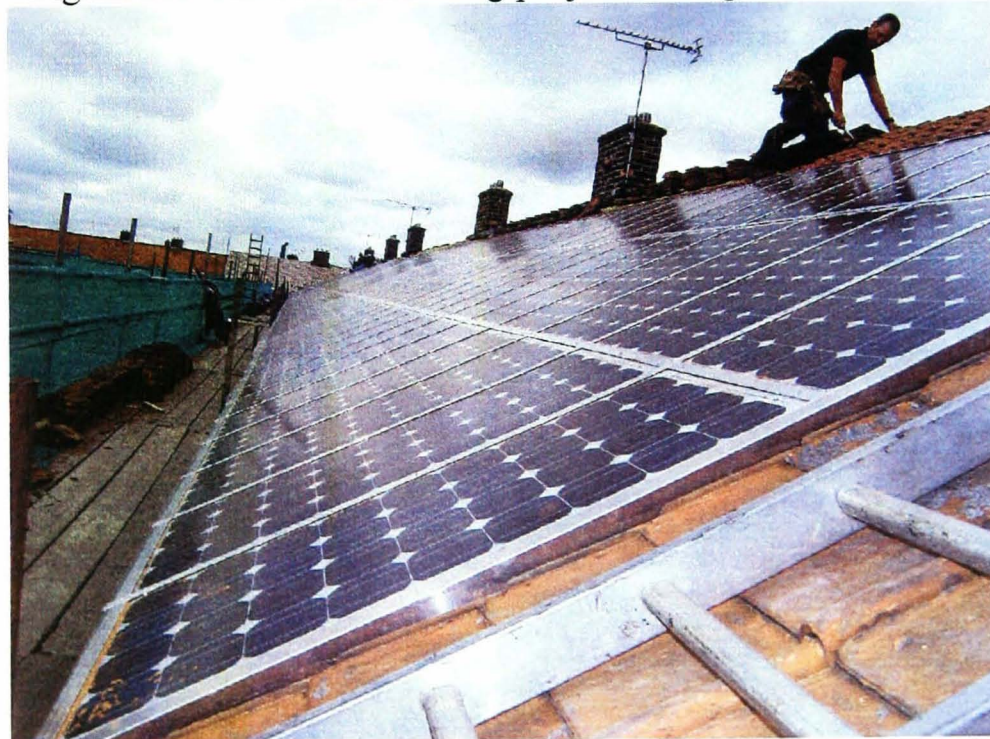
Figure 5.1 The social housing project during PV installation
