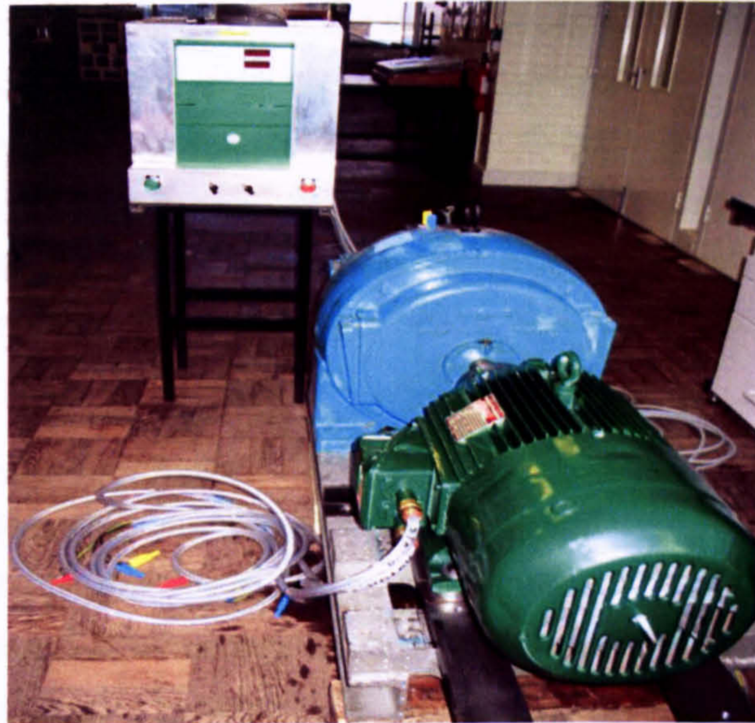
Figure D.4. Wind turbine simulator test rig motors
