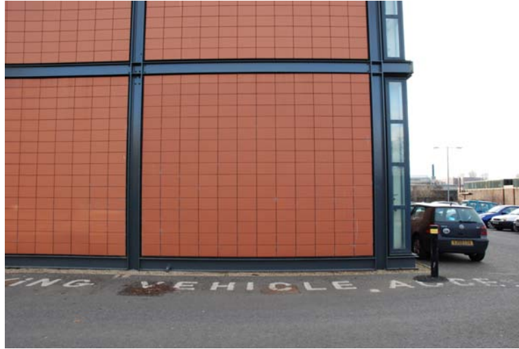
Figure 3.5: Outdoor plumb-line test field
