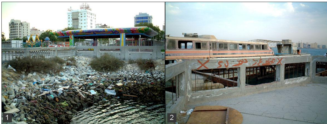
Figure 7.12: Bulkhead details and maintenance could hamper the level of interaction with the water, BC-I (December 2003)
