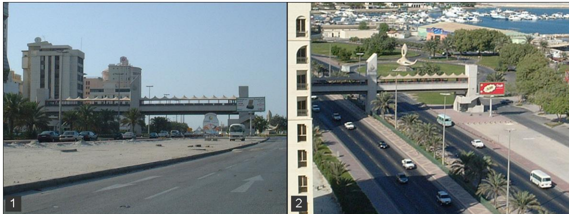
Figure 7.2: The Overpass on Al Fatih Highway (December 2003). (Source: the Author)
