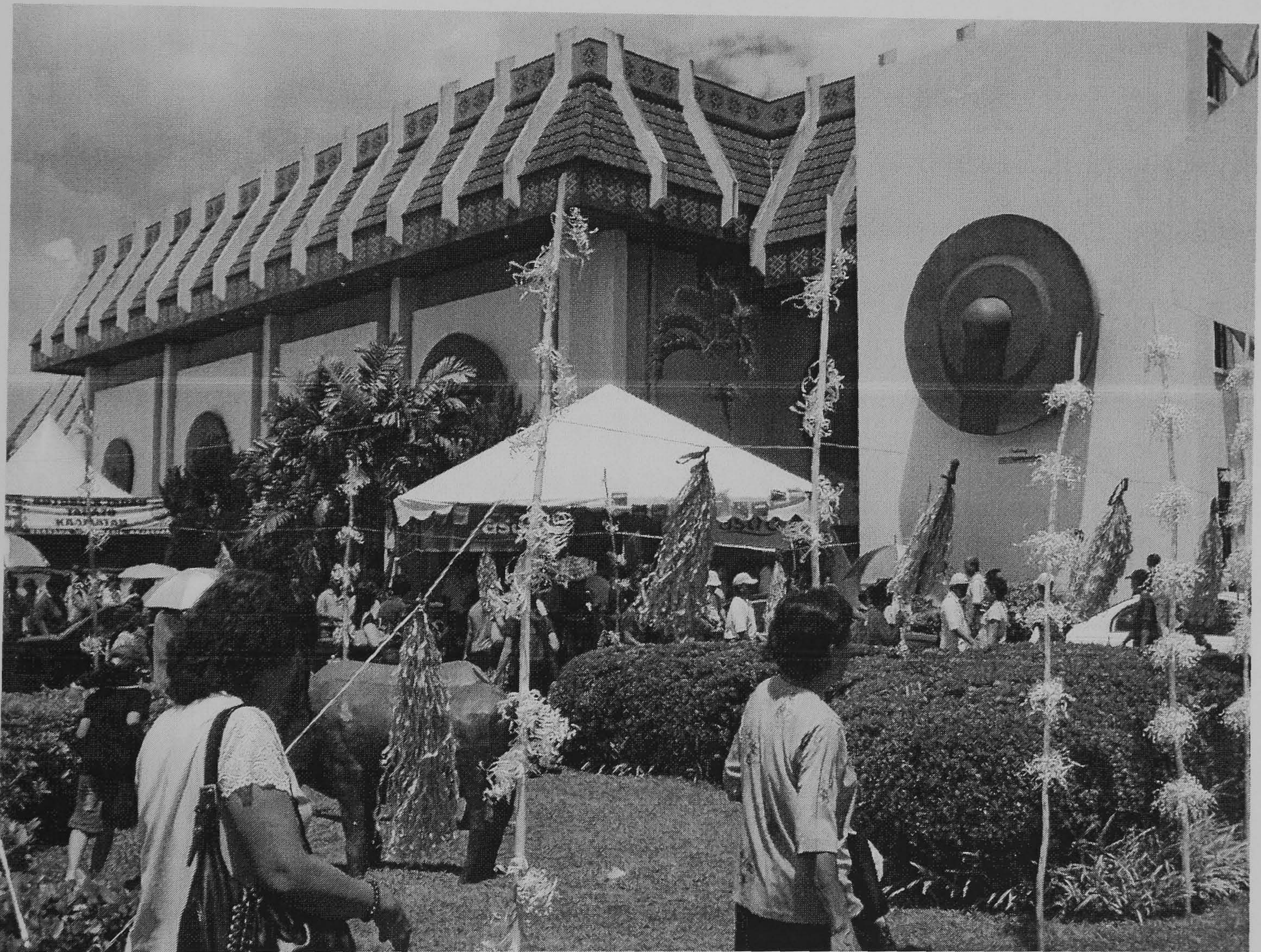
Figure 15 The side of KDCA main hall, built in a style re-elaborating traditional architectural designs; note the replicas of gongs, one of the symbols of Kadazan-ness, on the walls.
