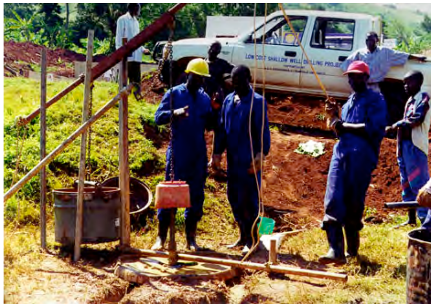
Figure 4.2: The First Pounder Rig in Operation
