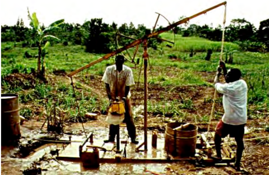
The Pounder Rig in Operation
