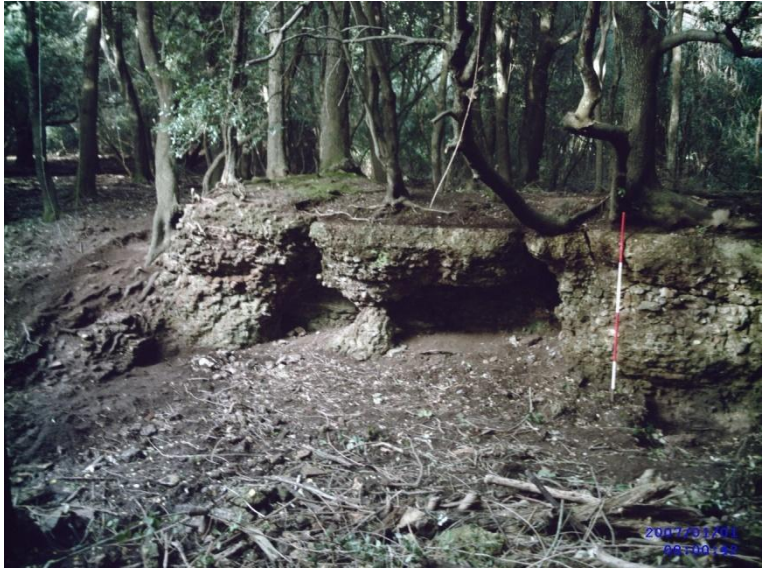
Plate 5.1: Sea wall looking north. Wave energy is concentrated heavily on the NW interior corner. The waterlogged depression in front of the wall is partially filled with aeolian sand and rubble. A small wave-eroded pillar is the only thing preventing the mid-portion of the wall from collapsing under the weight of the mature Holm oaks now growing out of the ornamental pond. The badly damaged NW mole (breakwater) is visible on the extreme left of the image as a low tumble of masonry delineated on the exterior face by extensive tree-roots.
