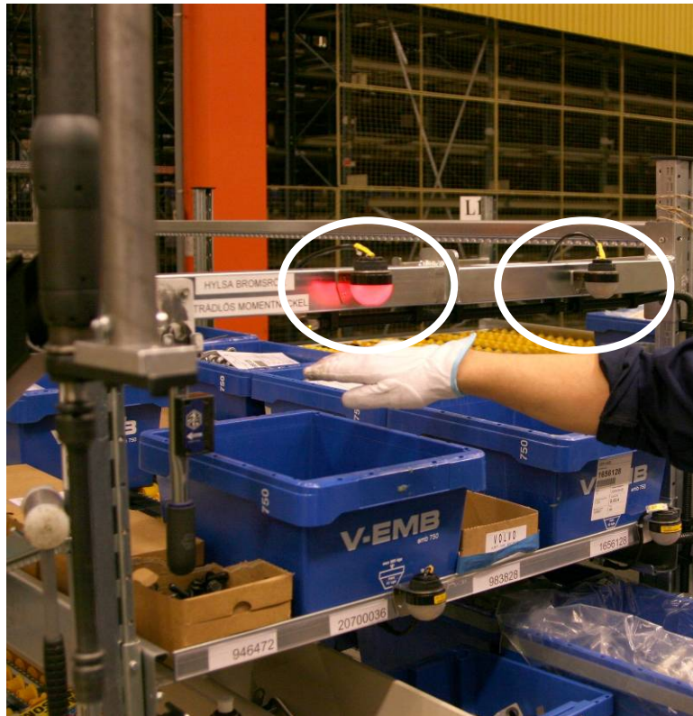
Figure 4.9: Light indicating what part to pick next. This specific installation includes a photocell that when affected, registers when a part is picked.
