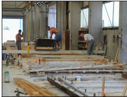
Figure 5.8 Offsite manufacture of precast panels; placing concrete in moulds
