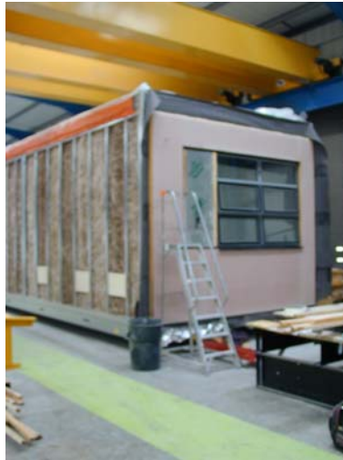
Figure 5.5 Offsite manufactured modular building
