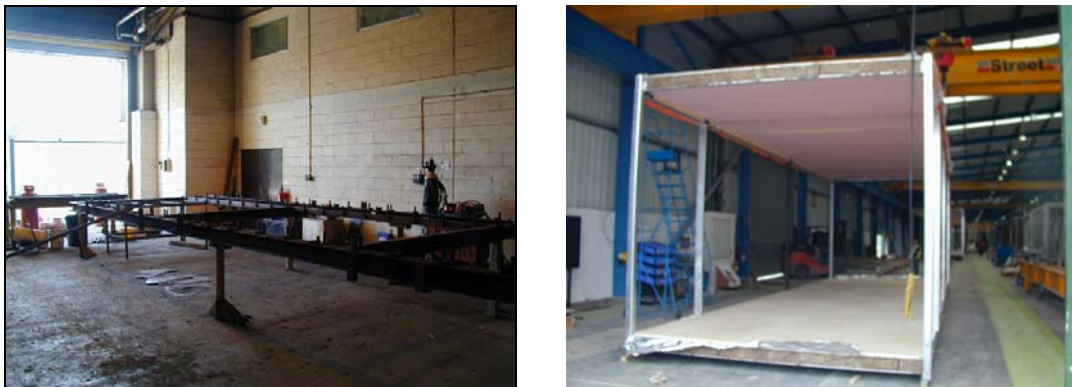
Figure 5.13 Modular building manufacture; floor cassette and wall elements
