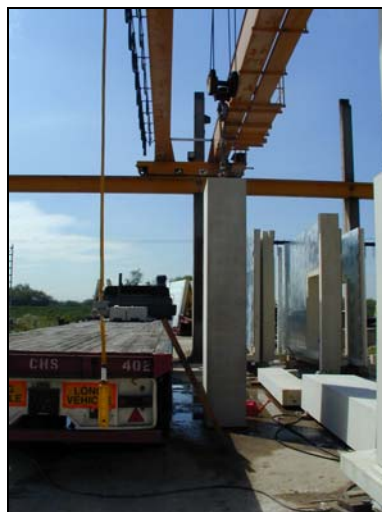
Figure 5.9 Offsite manufacture of precast panels; storage of units
