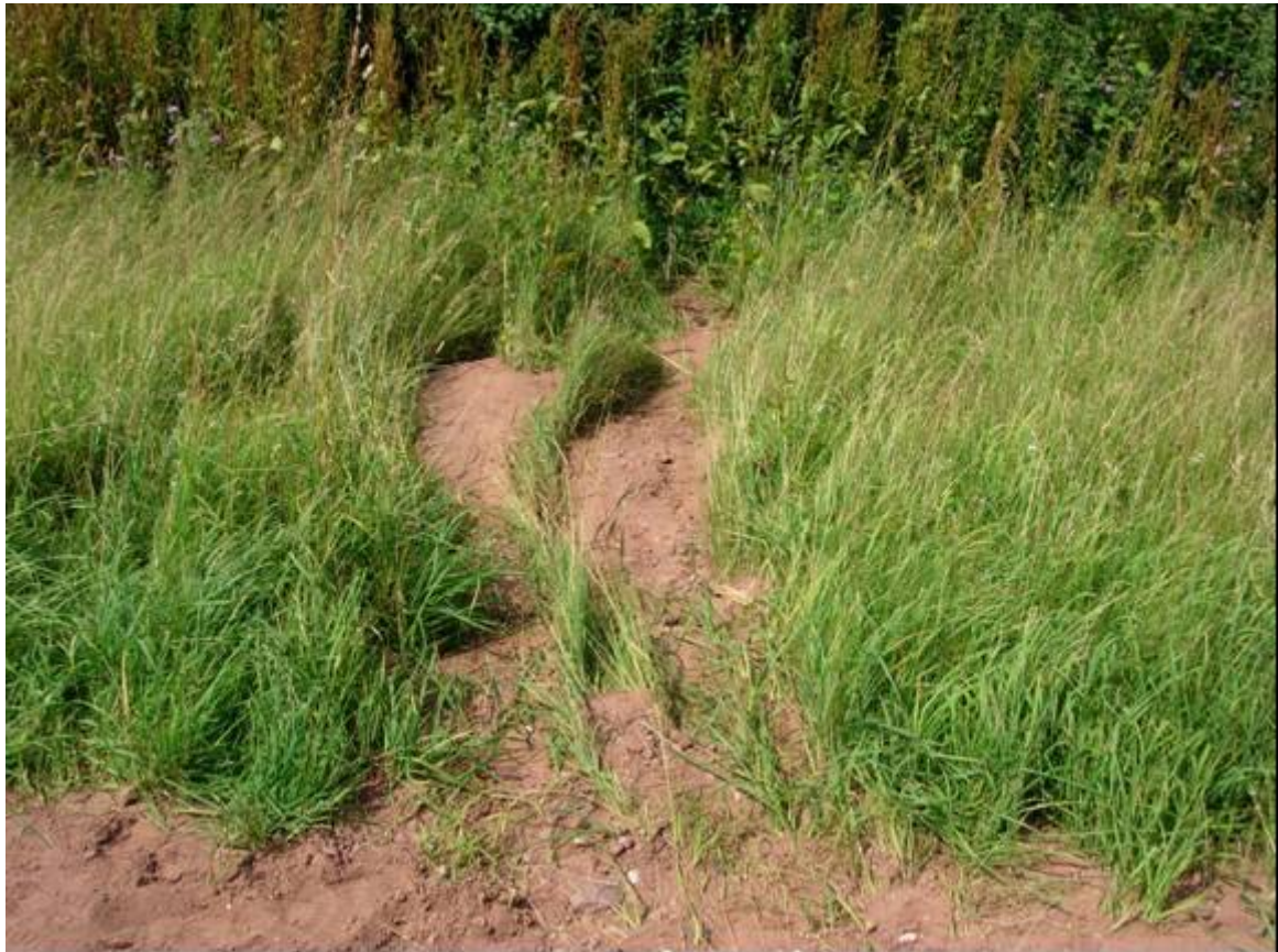
Figure 5.52 Breach points in the VFS at Site 9 caused by concentrated flow.
