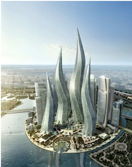
(a) Dubai Towers (construction on hold)
